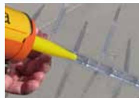
Glue troughs along the base make for easy installation. Bird-B-Gone offers construction grade adhesives.
