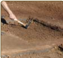
Excavate the batter's box 3" deep.
