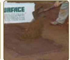
Cover with a 1/4" layer of infield mix to finish grade. Top entire home plate or mound area with Turface MVP or Pro League.
