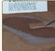
Apply a thin layer of Professional Mound Clay (match color to blocks) moisten, tamp.
