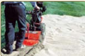
Rototill Field & Fairway into the soil at a rate of 1 to 2 tons per 1,000 sq ft.
