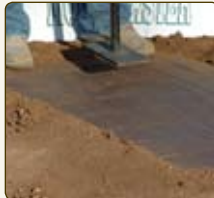
Install MoundMaster Blocks, moisten, tamp, then fully water and allow to soak in for 20 minutes.
